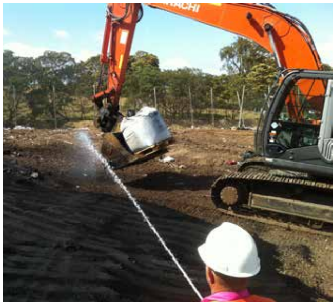
Adding RemBind to form the base of the burial pit
